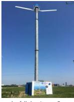
more capacity from the windmill compared to full electric ones. Excess wind energy is used to produce electricity and in combination with solar energy we create an off-grid micro network (if no electric grid is available). This can be used as well for periods of wind flaws. The fresh water can be used for irrigation, drinking water for animals or drinking water for humans.
